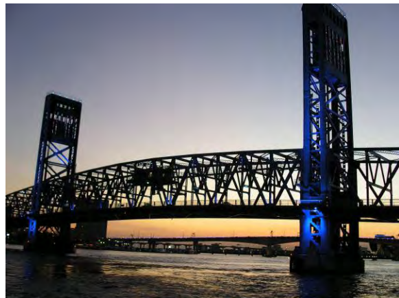
Main Street Bridge, over the Saint Johns River Jacksonville, FL.
